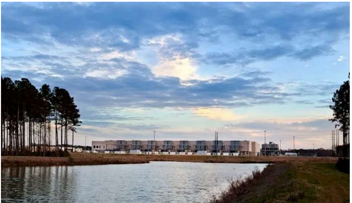
A Google data center in Berkeley County, South Carolina (Google)
