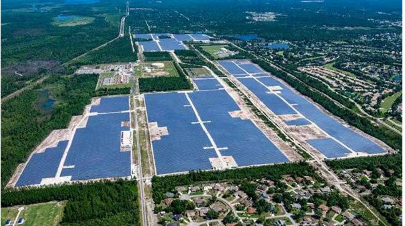
The DeBary Solar Power Plant in Volusia County, Fla., began serving customers on May 14, 2020. The facility is 74.5 MW with 300,000 panels. Courtesy: Duke Energy
